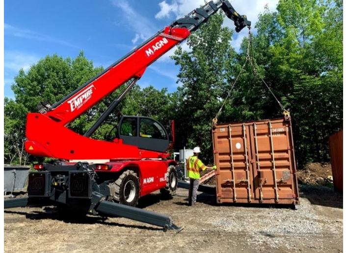
View of mobilized jobsite trailers after being unloaded from trailer.
