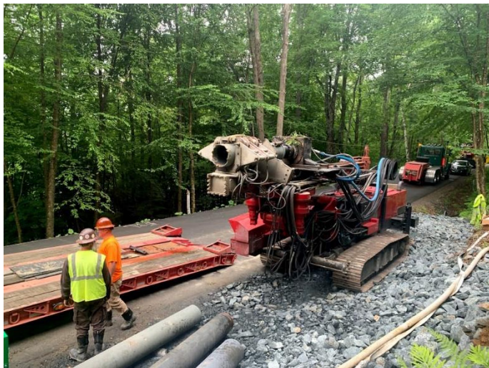
Offloading of Elletari MD 7000 drilling rig along Mine Road.
