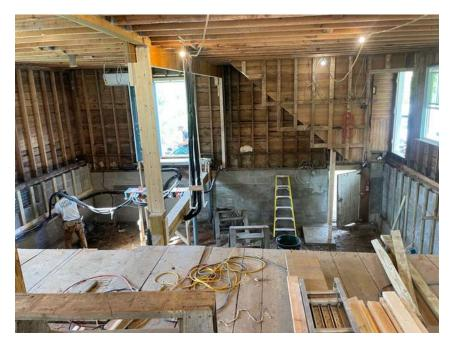
The scope of the work at the Strafford Historical Society Building includes a complete structural reworking of the first floor and cellar.
